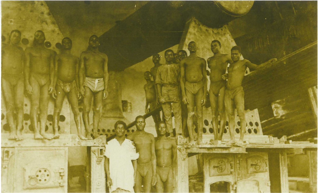
77. Skupinski posnetek domačih delavcev po uspešni namestitvi parnih kotlov. / Photograph of a group of native workers after successful installation of the steam boilers.
